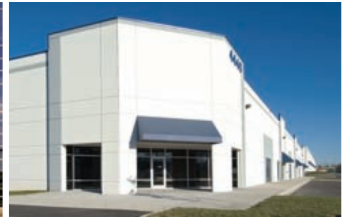
Federal Emergency Management Agency Wedgewood South – High Bay Warehouse
